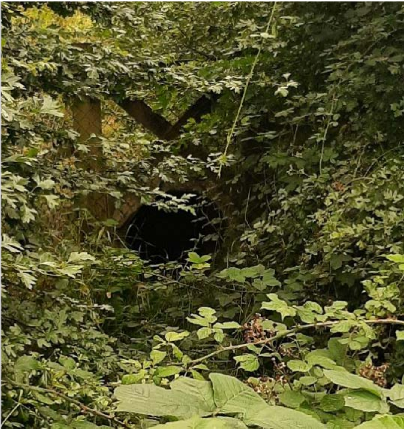
Figure 14.18. View of the 600m culvert (possible mammal underpass) taken from the eastern side of the R157 near the gap in the fence.
