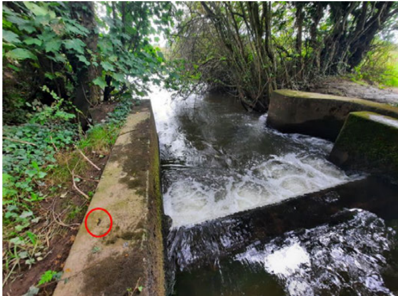
Figure 14.24. Location of spraint in red, recorded along a concrete weir structure.
