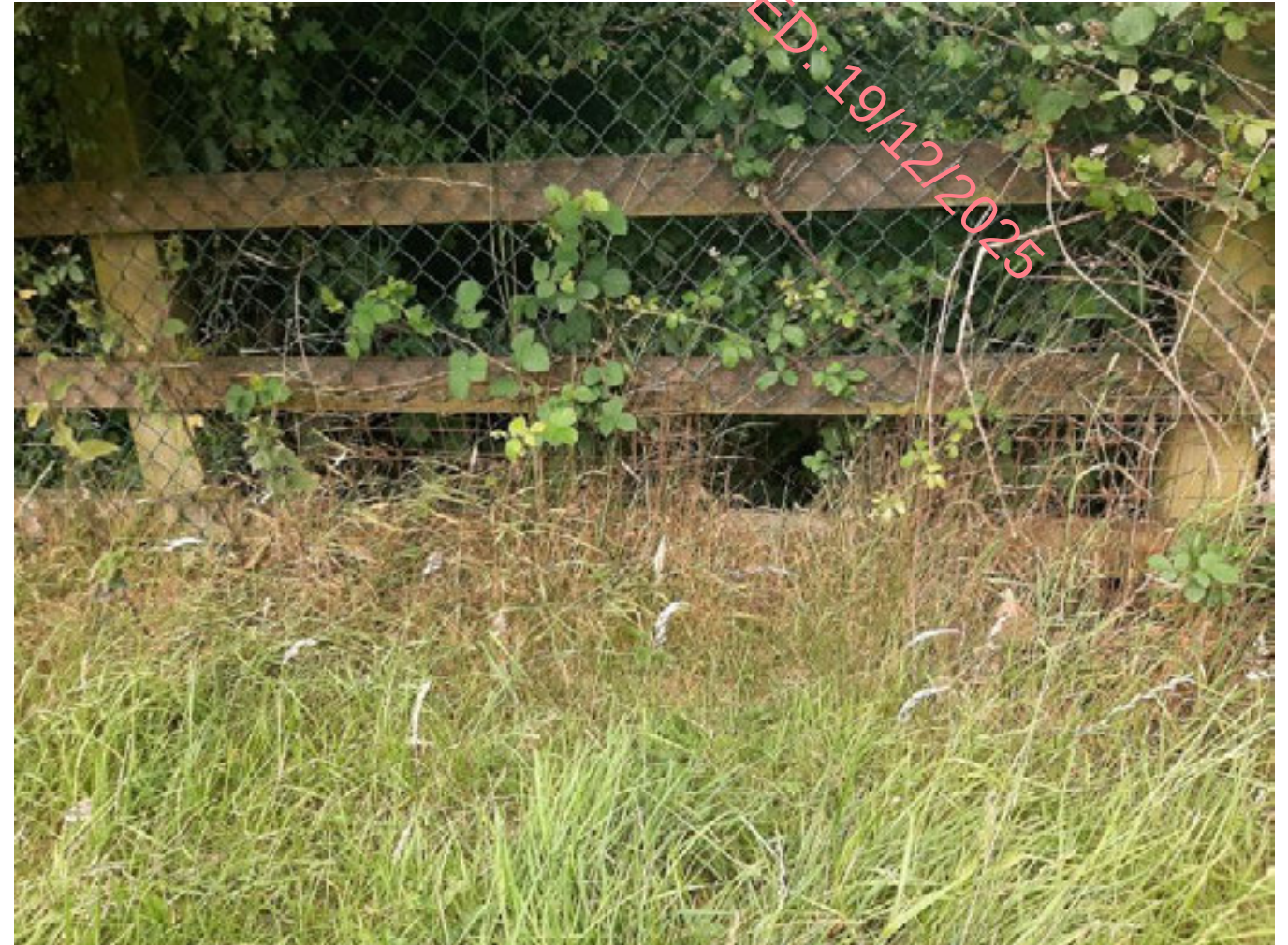
Figure 14.17. Manufactured gap in fencing located on the eastern side of the R157
